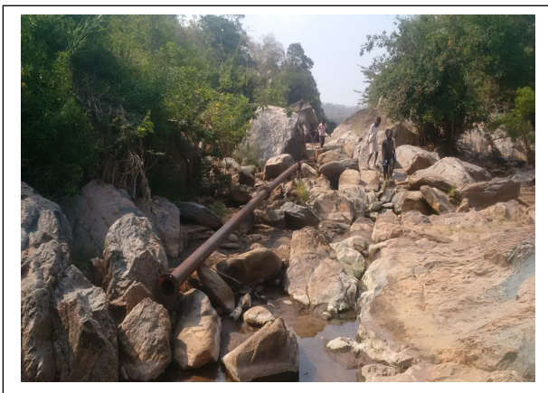
New Intake silted and abandoned
