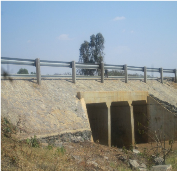
Three Cell Box Culvert near Bunda Junction
