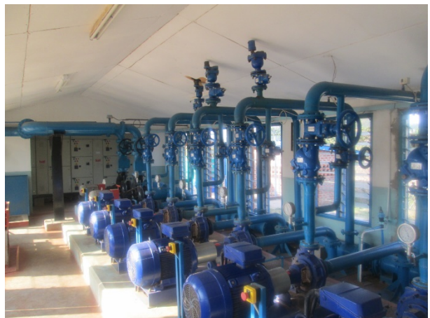
Pumps at Water Treatment Plant
