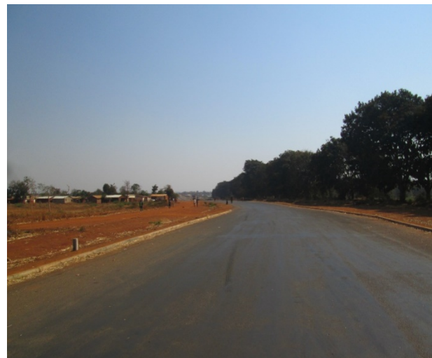
Completed Section near Mchinji Road Junction
