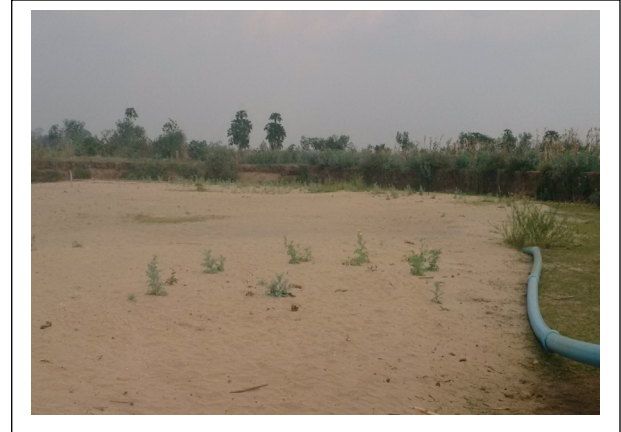
Main pipe washed away at Chapananga
