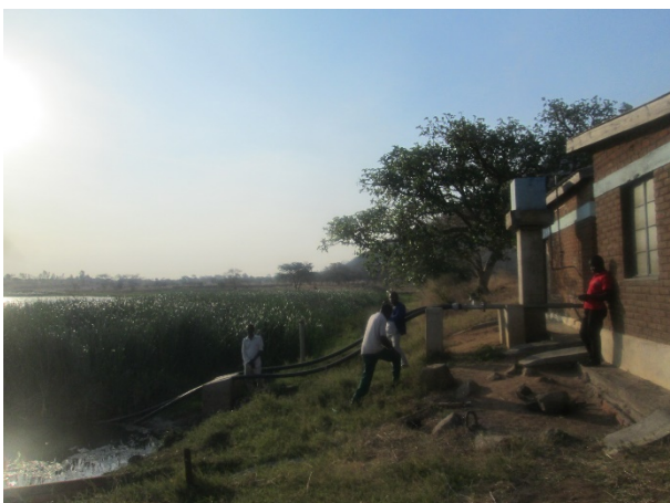
Nguluyanawambe Intake Pump House
