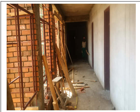
Internal Finishes of the Works
