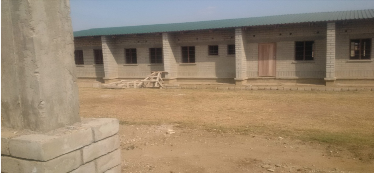
Machinga Secondary School – Incomplete Classrooms
