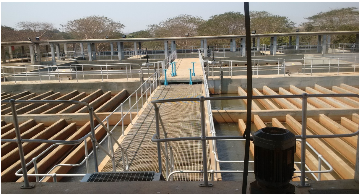
The New Lilongwe Water Board Treatment Works II
