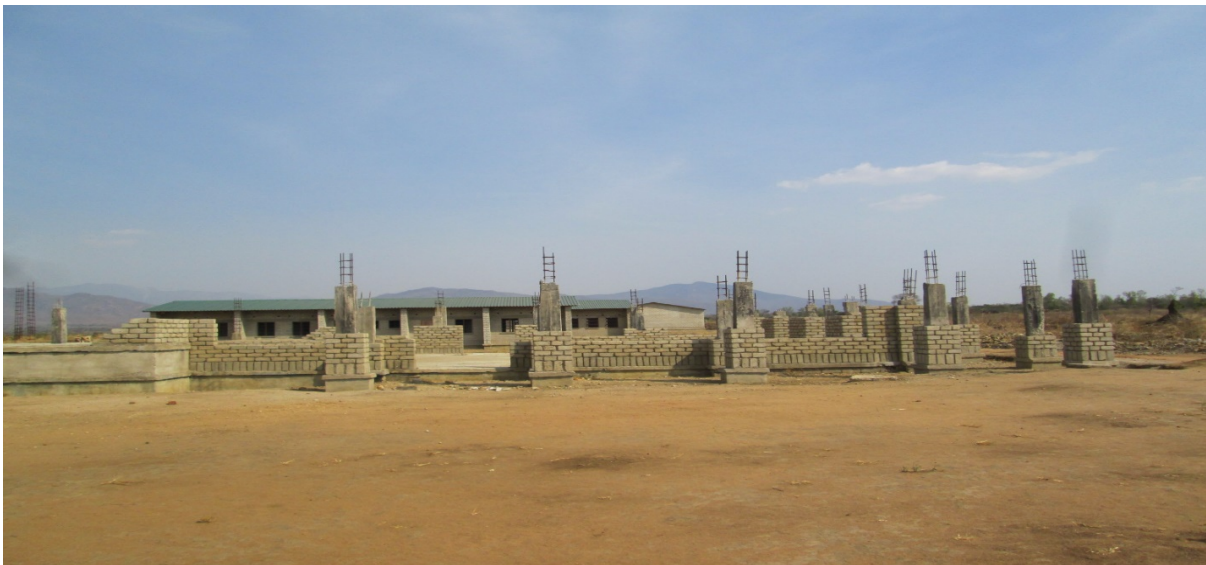
Machinga Secondary School – Incomplete and abandoned Administration Block
