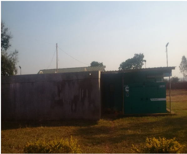
T2 Pumping Station Stand-by Generator & Tank
