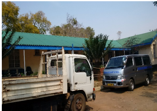
Administration Block – Rehabilitation
