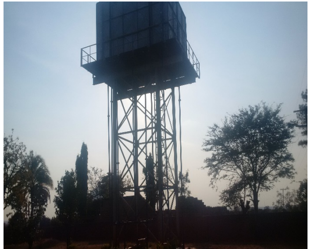
T2 High Level Supply Tank
