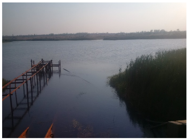
Nguluyanawambe Intake Structure
