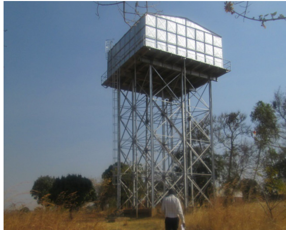
High Level Distribution Tank
