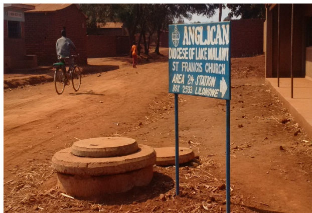
Valve Chamber at Area 24
