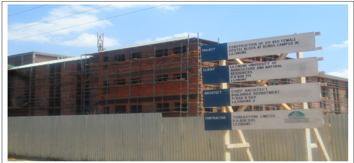
Project Sign Board – Public Disclosure of the project
