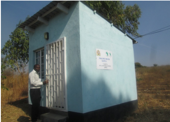
Malomo Water Supply - Pump Switch Room
