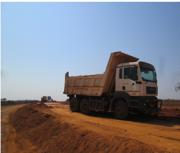
Earthworks in Progress
