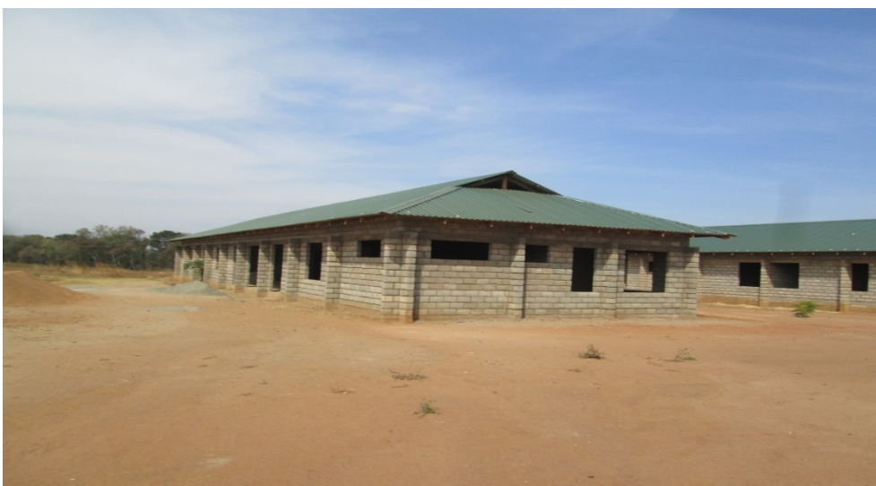
Domasi Rural Hospital Project – Abandoned incomplete Buildings
