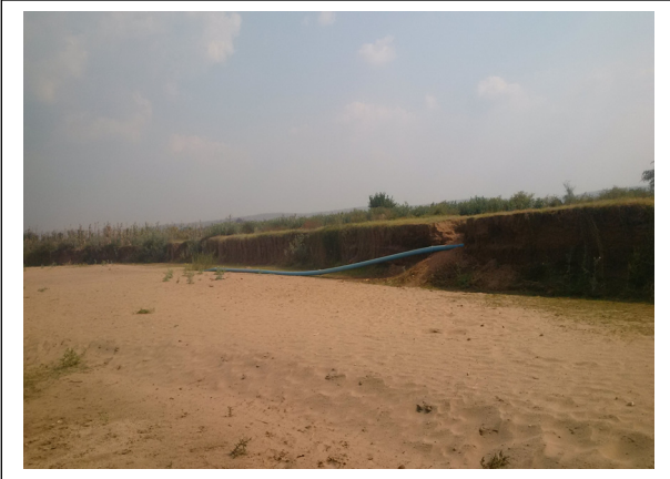
Main Pipe washed away at Chapananga
