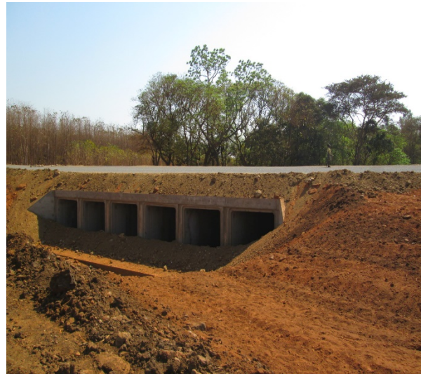
Six Cell Box Culvert
