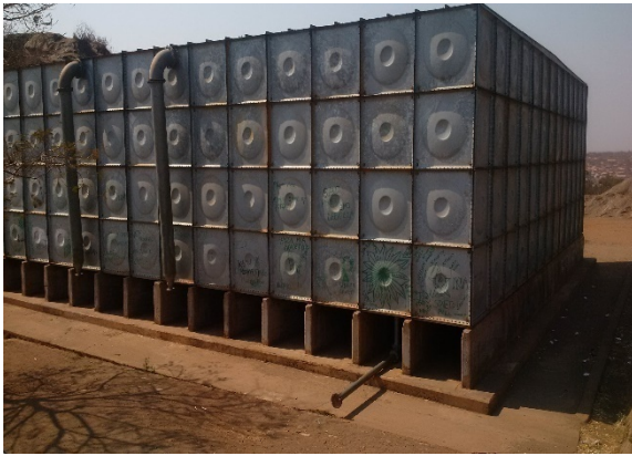
Refurbished water tank at Ngwenya
