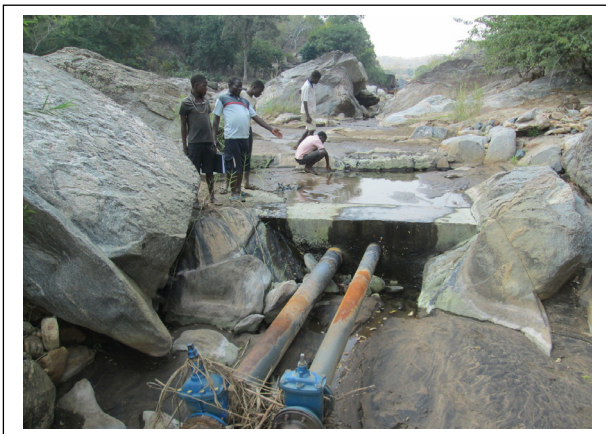
New Intake silted and abandoned
