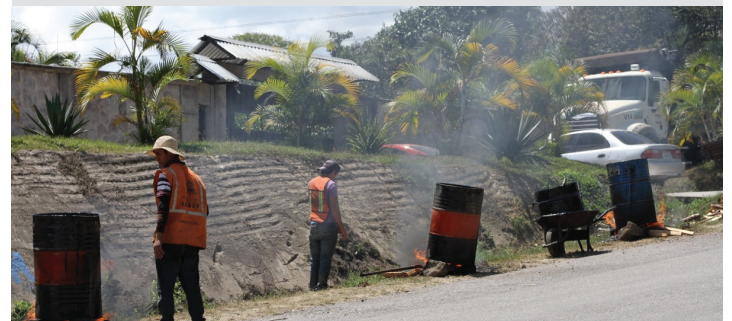
Burning of asphalt in open containers during a road maintenance project from Siguatepeque to La Esperanza.
