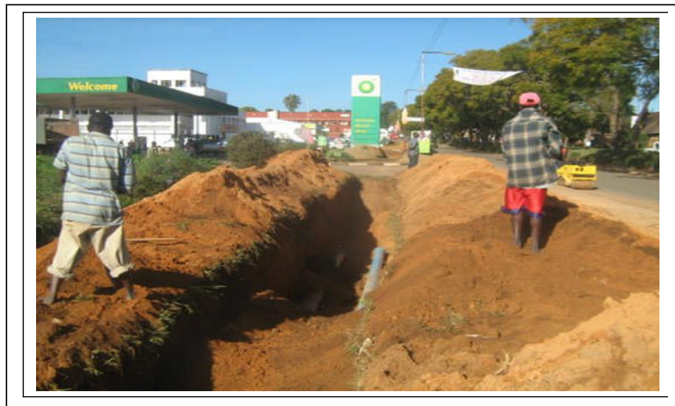
NRWB 1 – Labourers wearing no protective gear; no warning signs; no marker tape
