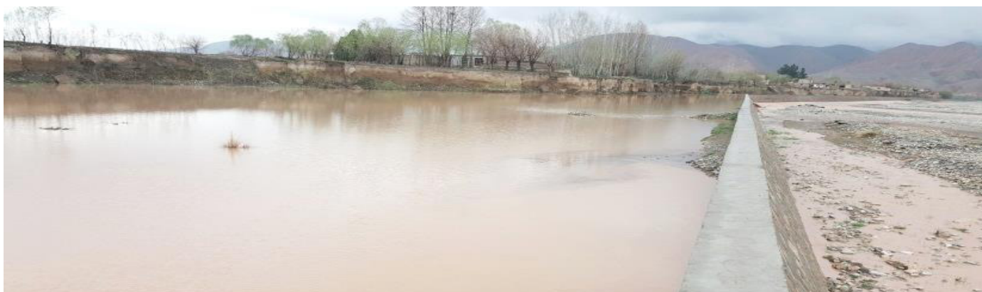
Water Ponding Behind the Retaining Wall
