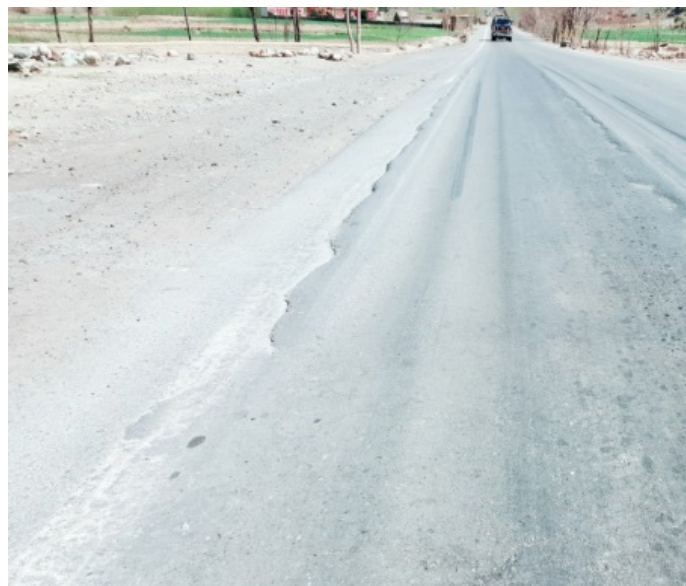
Rutting of the Pavement Surface
