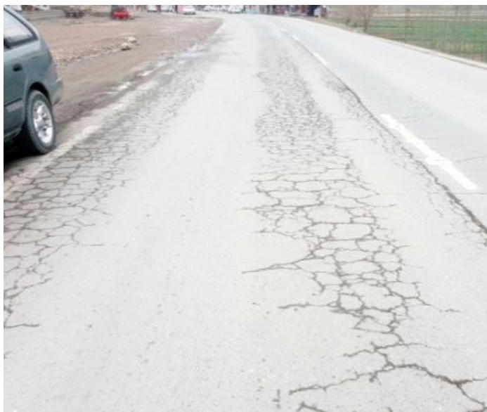
Cracks on Surface of the Road
