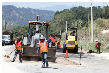
Road construction project assessed by the CoST Honduras Assurance Team.
