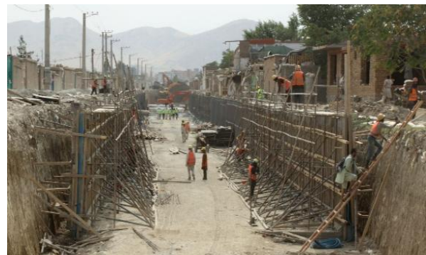
Figure 26: The project is under the formwork and steel work on section 4+430
