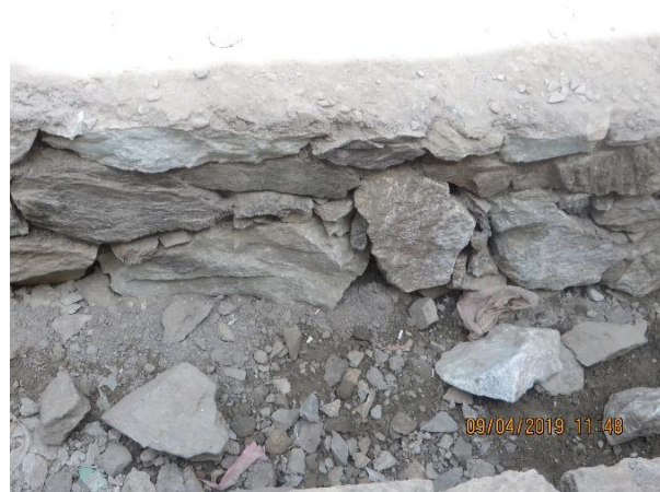
Figure 28: Improper stones and masonry observed at the site ditches
