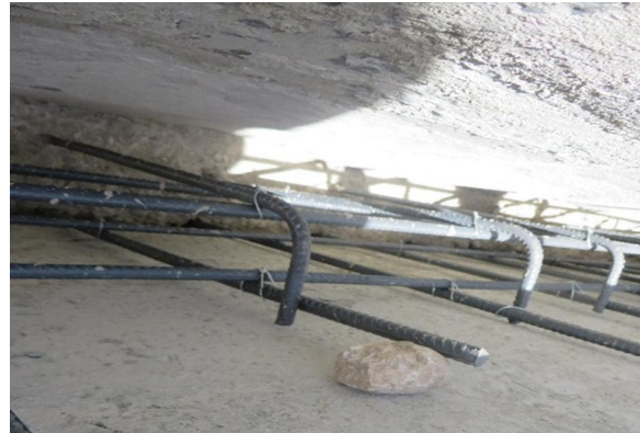
Figure: 12 No proper and sufficient spacers were used between steel bars and formwork of the ditches
