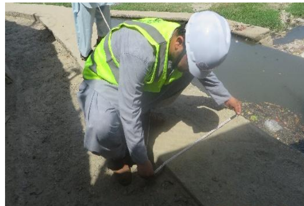
Figure 16: CoST AT is measuring the project specific items
