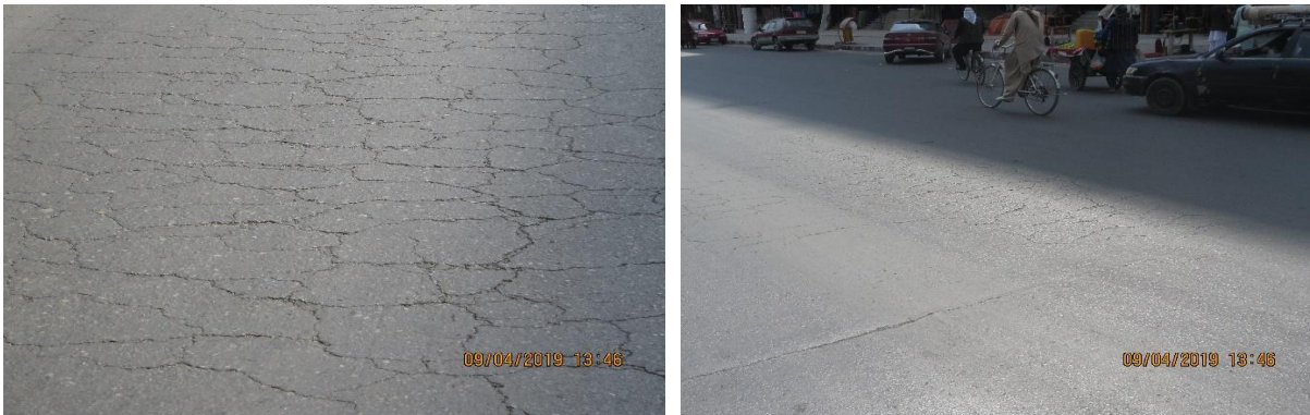
Figure 29: critical cracks (crocodile / fatigue) are visible along the whole length of the road while the project is on the second year of construction
