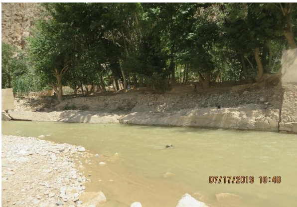
Figure 17: due to recent flood part of the protection scheme were damaged on location 0+00 of the project
