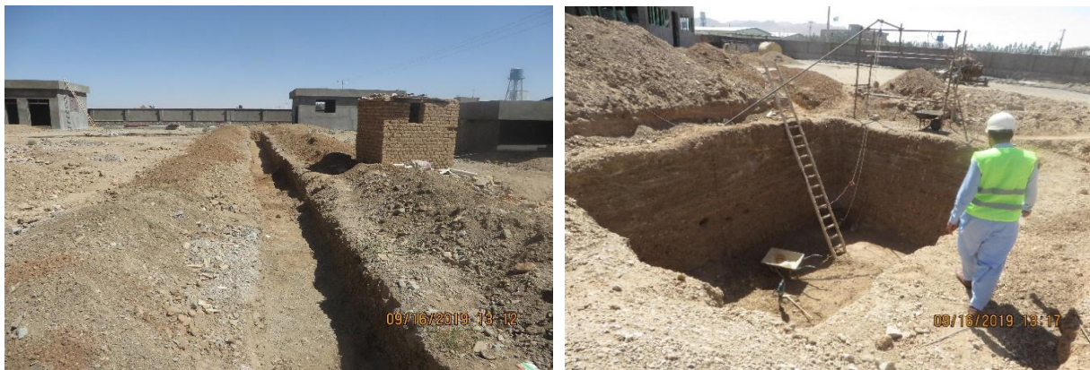
Figure 24: No warning tape was not used around the excavated ditches and septic tank
