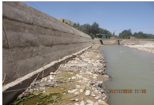
Figure 18: poor formwork was observed throughout the scheme wall
