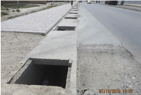
Figure: 11 Steel grating ditch covers were not installed where the construction of ditches culverts completed
