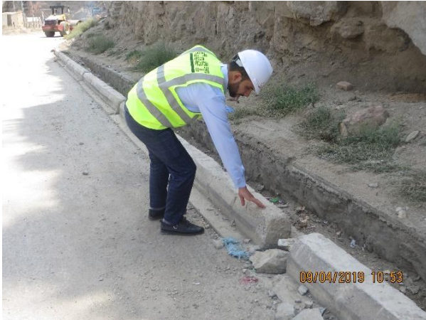
Figure 27: Concrete peelings were observed at the surface of installed curbstones
