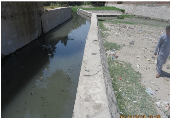
Figure 15: 15 cm thick PCC is peeled on section C-C of Canal which might cause from improper curing during the construction
