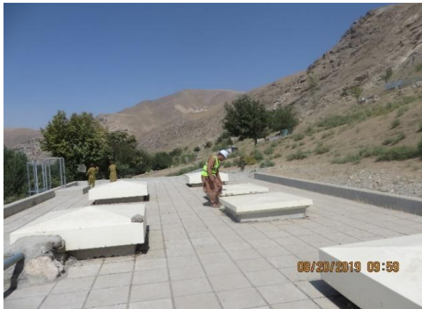
Figure 19: CoST AT is visiting the project. No protection walls have been considered.
