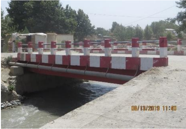
Figure 13: Construction of 12-meters Concrete bridge, Takhar Province
