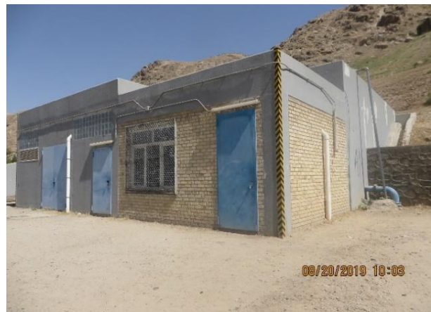
Figure 20: No person has been appointed for the maintenance of the project
