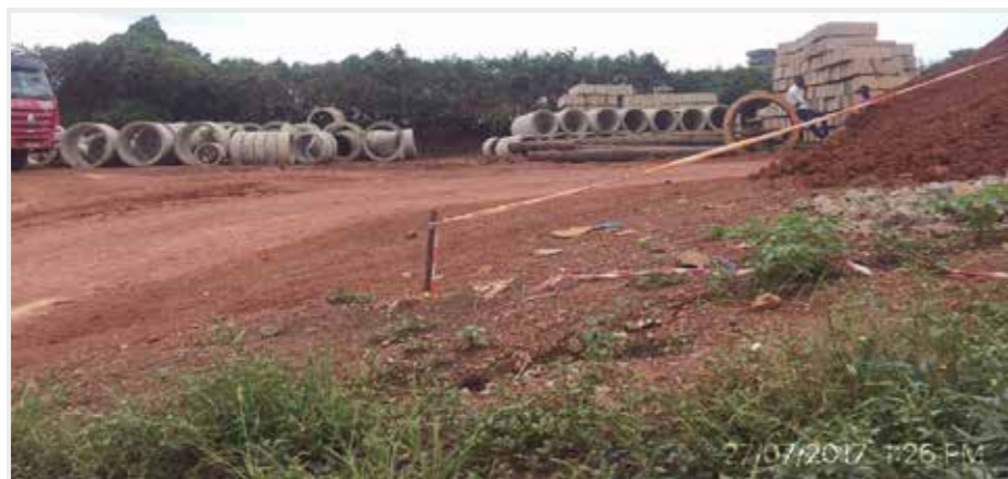
Figure 15: Stoke pile area unsecured
