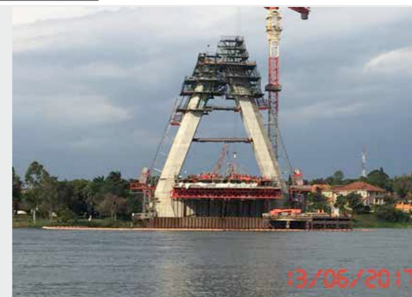
Figure 41: New Nile Bridge under construction
