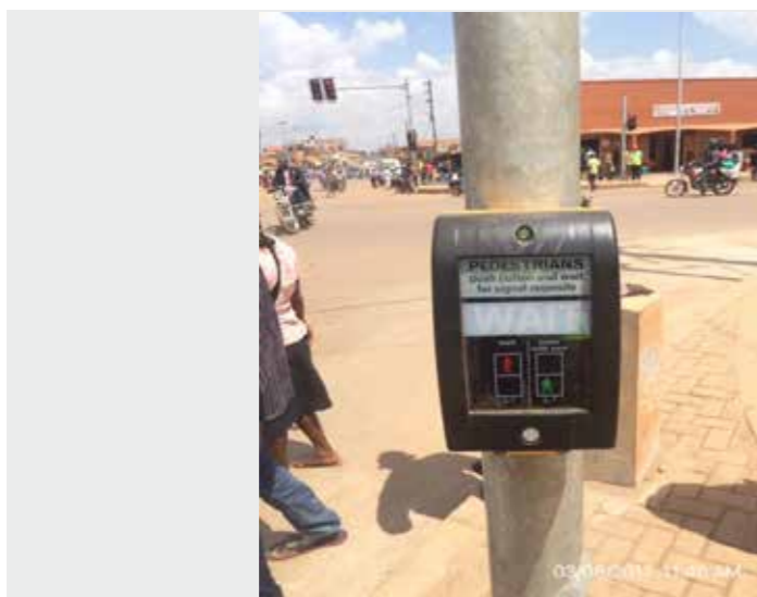
Figure 31: Pedestrian push button signal
