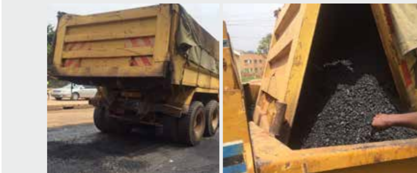
Figure 18: Truck offloading asphalt in the paver
