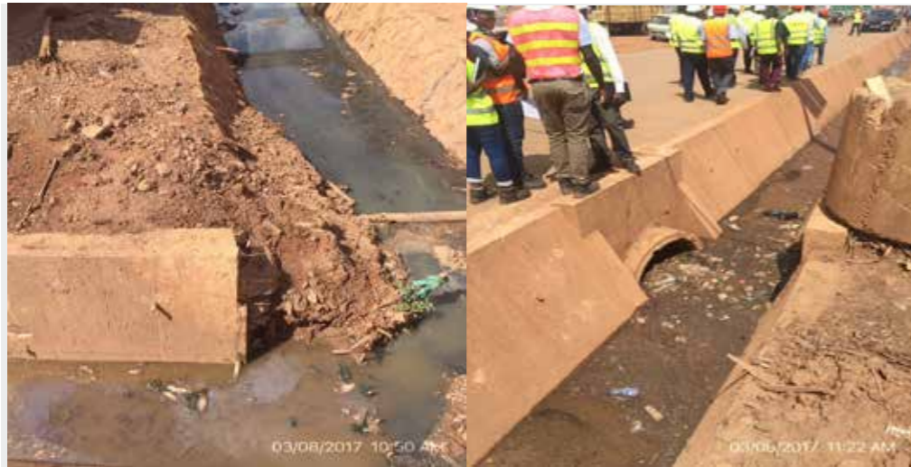
Left – Right: Figure 35: Uncompleted Side walls Figure 36: siltation and wastes
