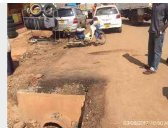
Figure 33: Access road with 2m but with unprotected shoulder
