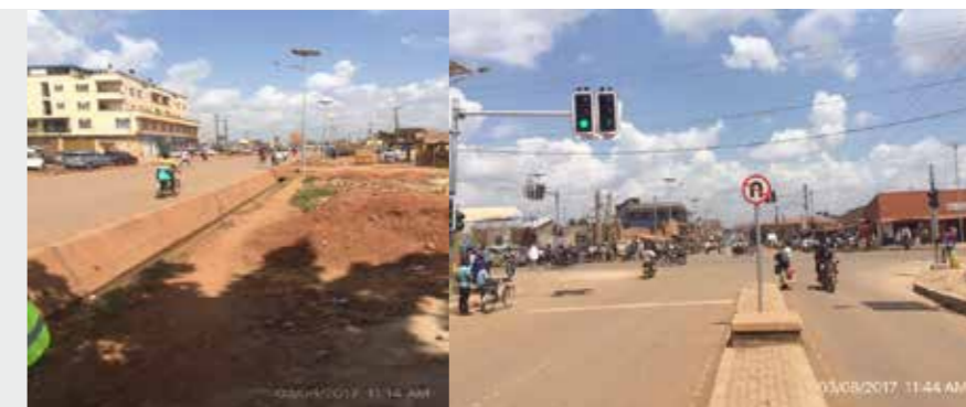
Figure 32: Traffic lights and street lights
