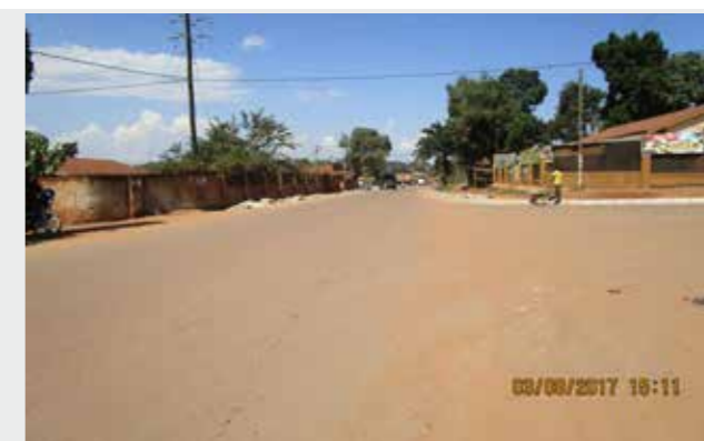
Figure 11: Showing completion status of Sembera road – no completion data disclosed.
