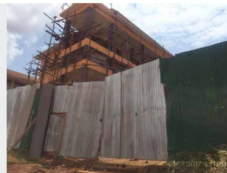
Figure 25: Makerere college block constructed under compensation funds
