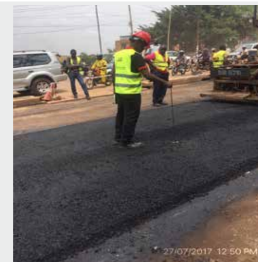
Figure 16: AP using a gauge to confirm the thickness (65mm) at km 0+150m
