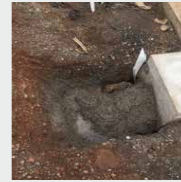
Figure 20: Uncompacted concrete as backfill
