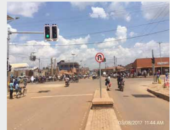
Figure 29: Road furniture (signs) provided
