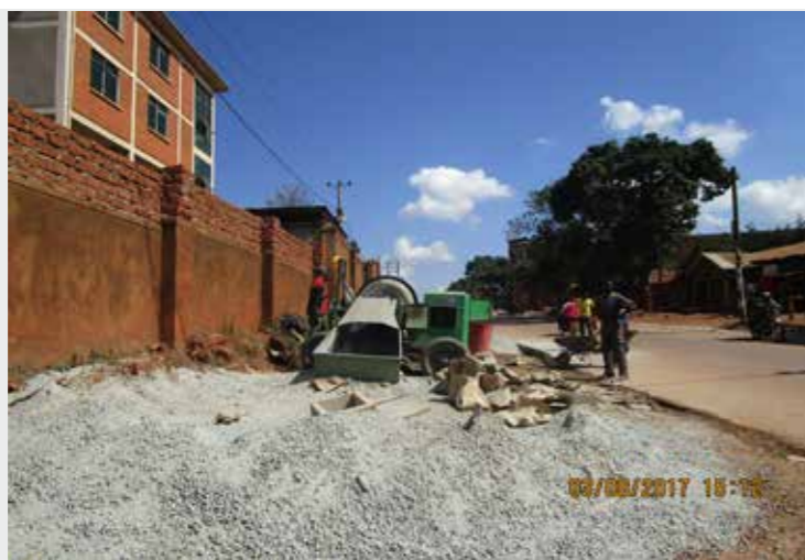
Figure 9: Concrete mixing for concrete works
