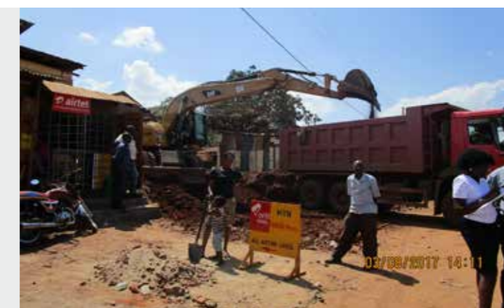
Figure 6: Removal of debris from construction site
