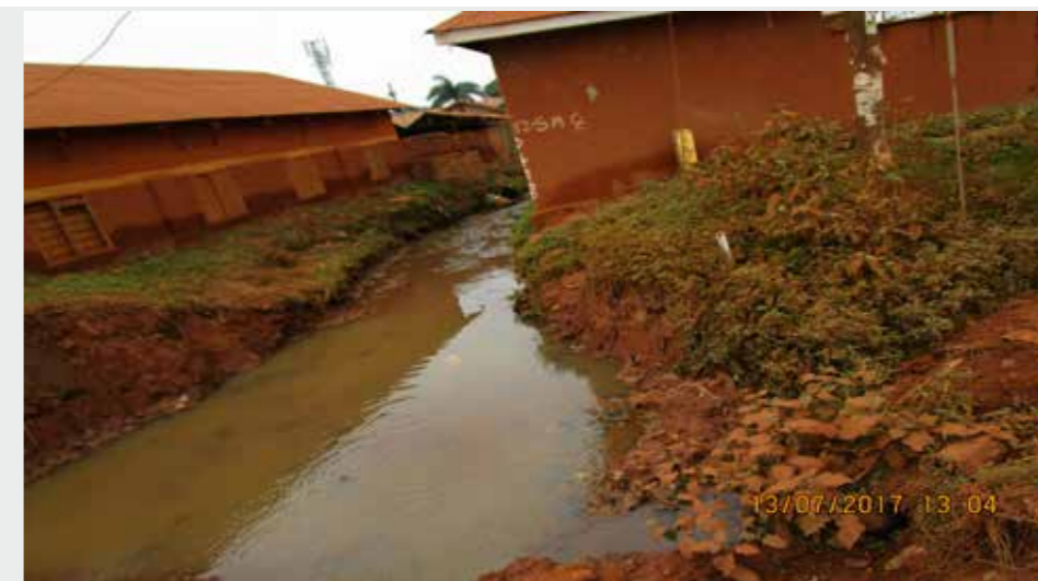
Figure 54: Outflow of water blocked by buildings.
