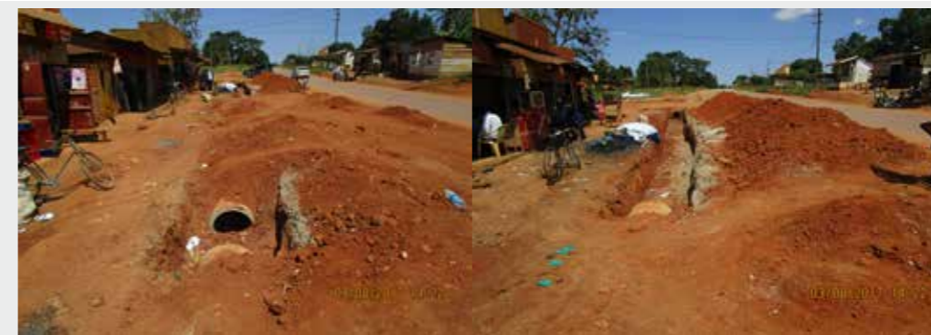
Figure 3: Construction of covered drains in progress along Gayaza road.
