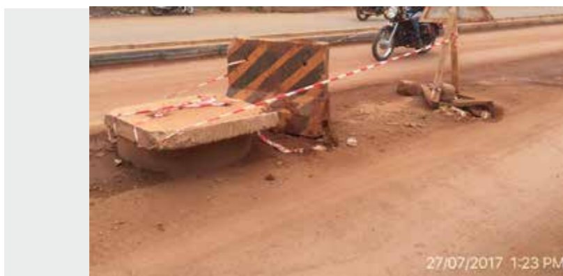
Figure 23: Culvert through the surface
