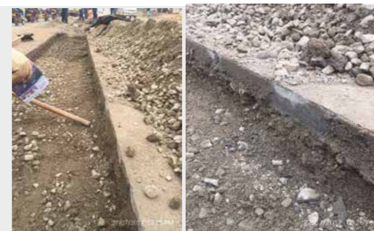
Figure 17: Asphalt Layer thickness (51mm) at km 0+020m
