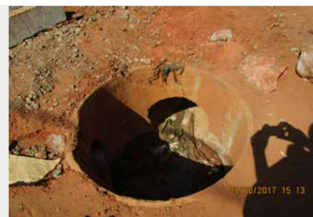
Figure 12: Construction of manhole for covered drains
