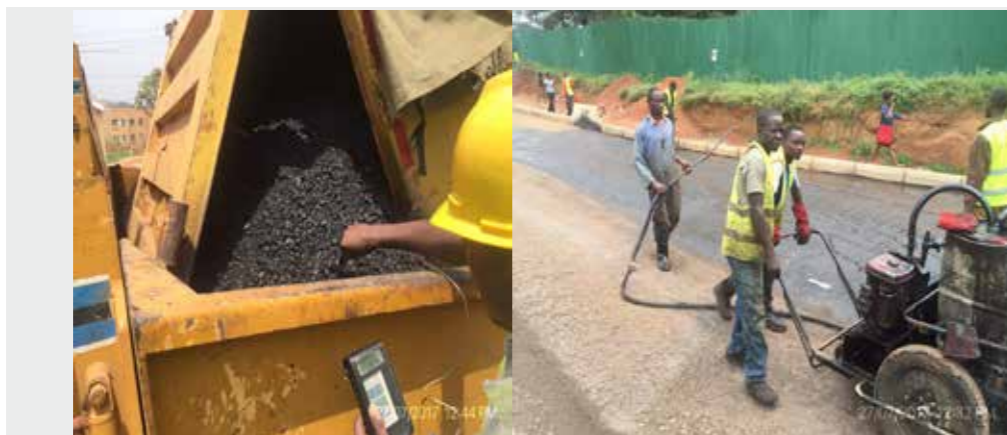
Figure 22: Safety issues at the site
