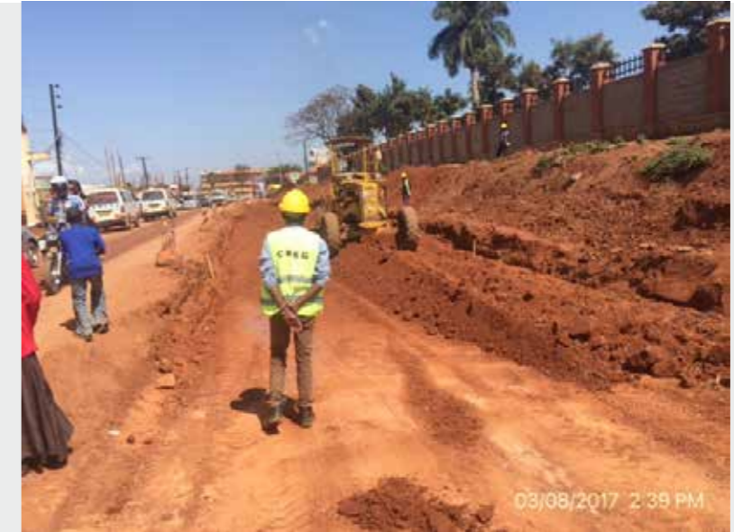
Figure 38: Contractor preparing subbase
