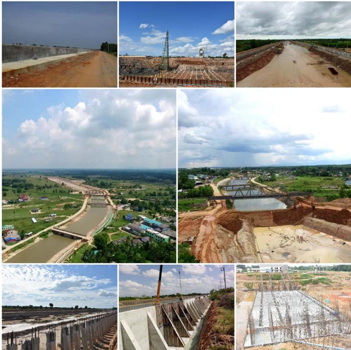
Figure 10: Progress on the construction of the flood relief project at Hat Yai (Phase 2), Songkhla province, Royal Irrigation Department
