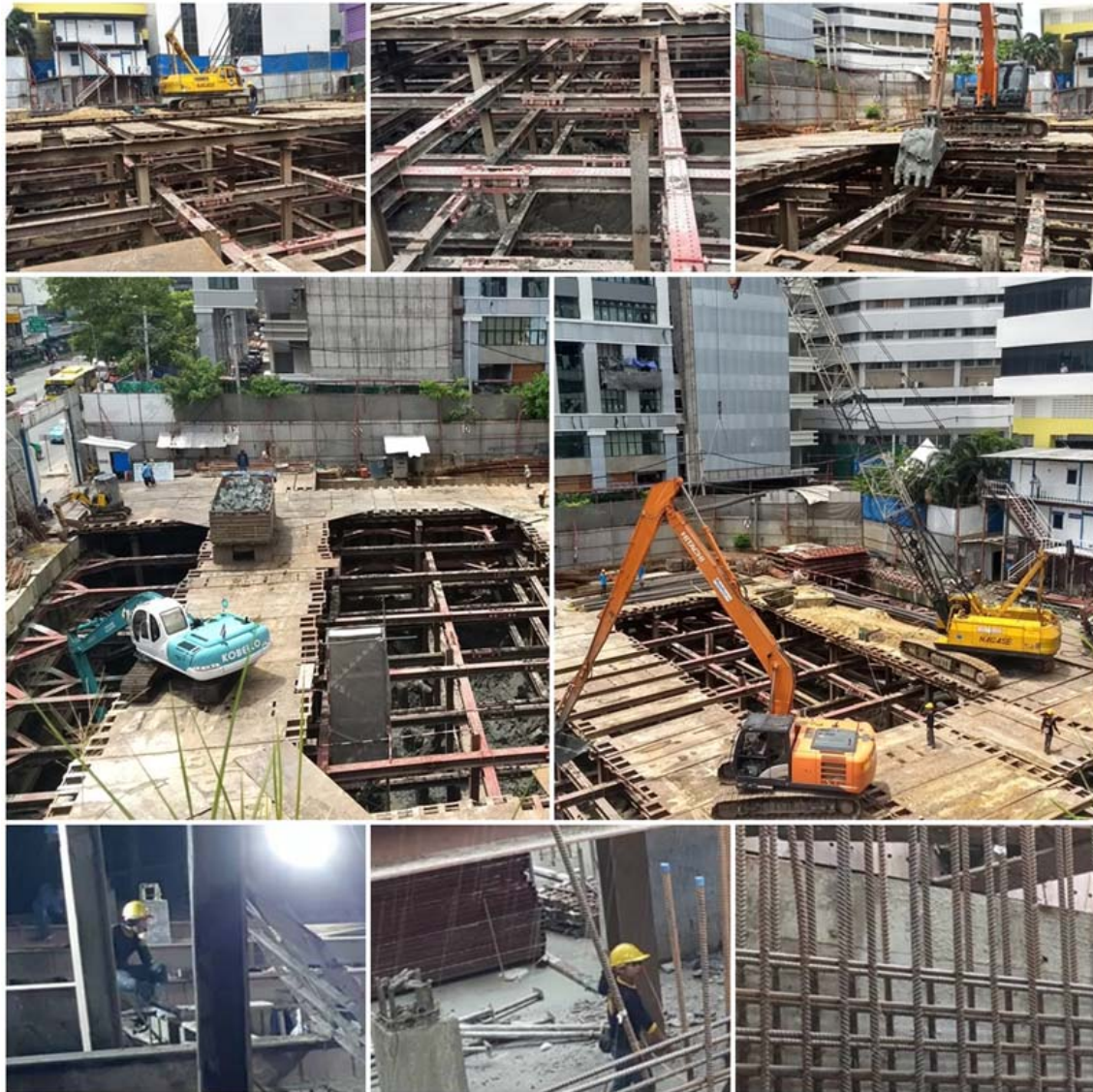
Figure 12: Progress on demolish and reconstruct the Institute of Dermatology building.
