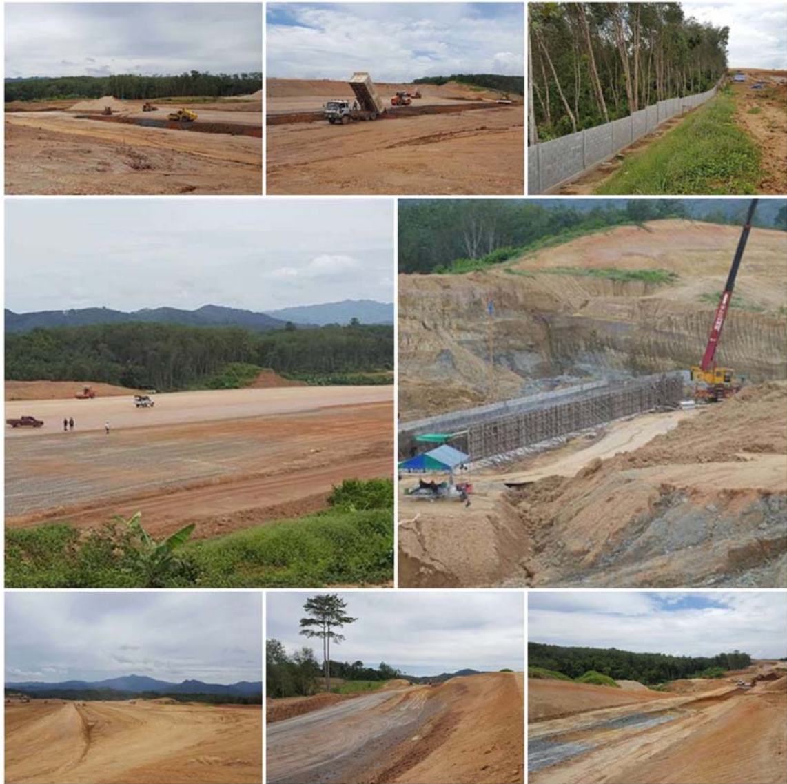
Figure 11: shows construction progress of runway, taxi way, apron, and etc. at Betong airport, Yala province, Department of airports.
