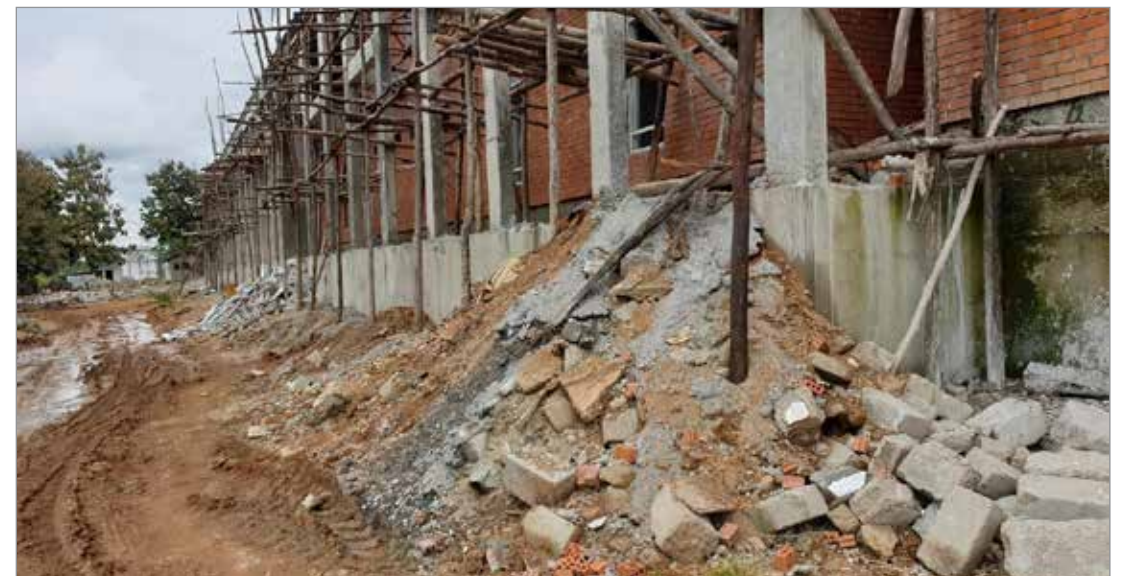
Debris piled on site and access road not maintained-Yumbe Project
