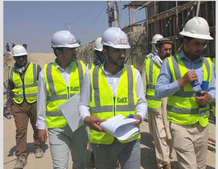
CoST Afghanistan Assurance Team on a site visit
