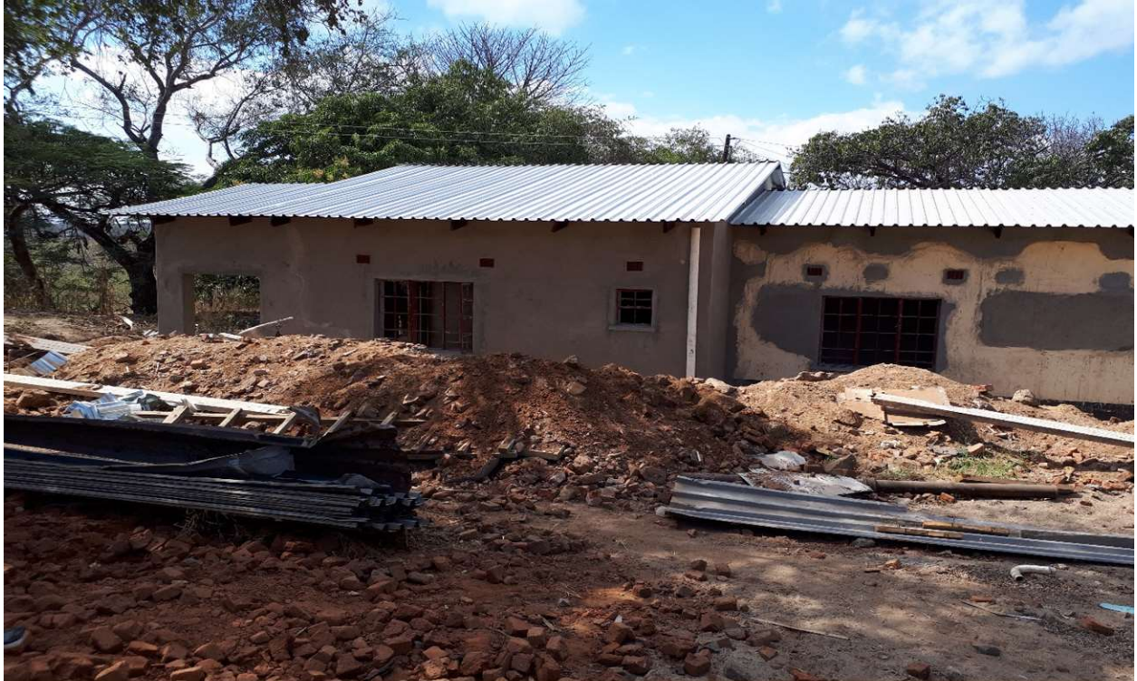
Picture 4.5.2.3 – Artisan 3 Bed Mapolisi Type House under Renovations
