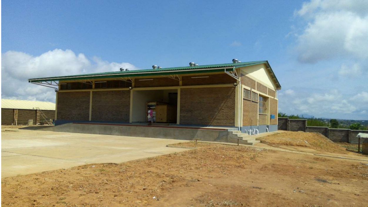
Picture 4.2.3.3 – Picture Showing the Cold Room Facility Externally
