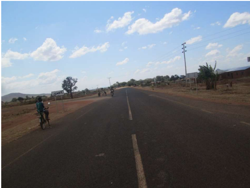
Picture 4.4.2.1 – Section of the Road near Jenda
