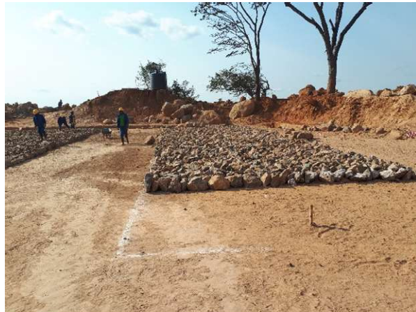
Picture 4.10.4 – Water Tank Foundations at Kazomba Hill
