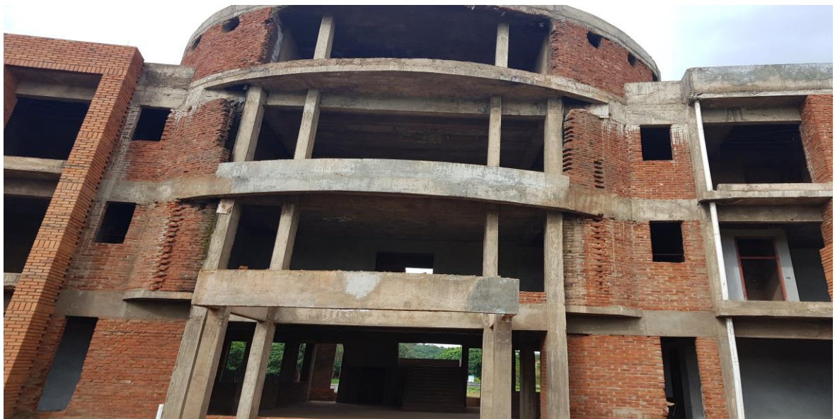
Picture 4.3.5 – Close-up View of Gateway Administration Block
