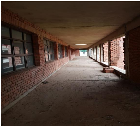
Picture 4.3.2 – Elevated Walkway
