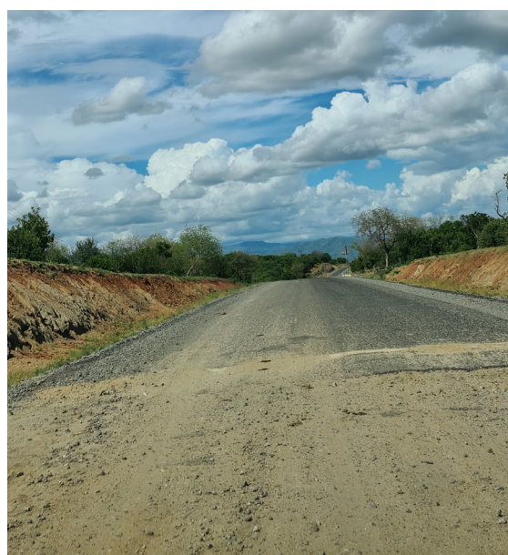
Photo 5 - Chikwawa Chapananga Road (End of Tarmac)
