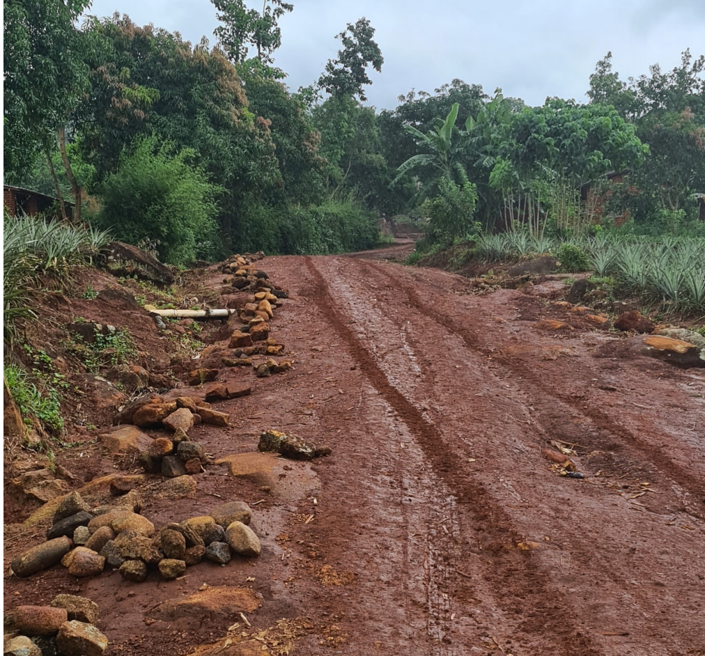
Photo 12 – Steep slippery Slope without Gravel
