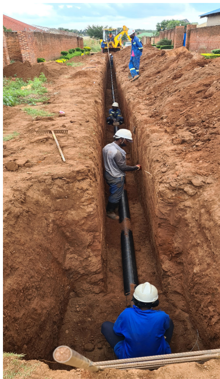
Photo 10 - Laying Sewer Line in Area 49
