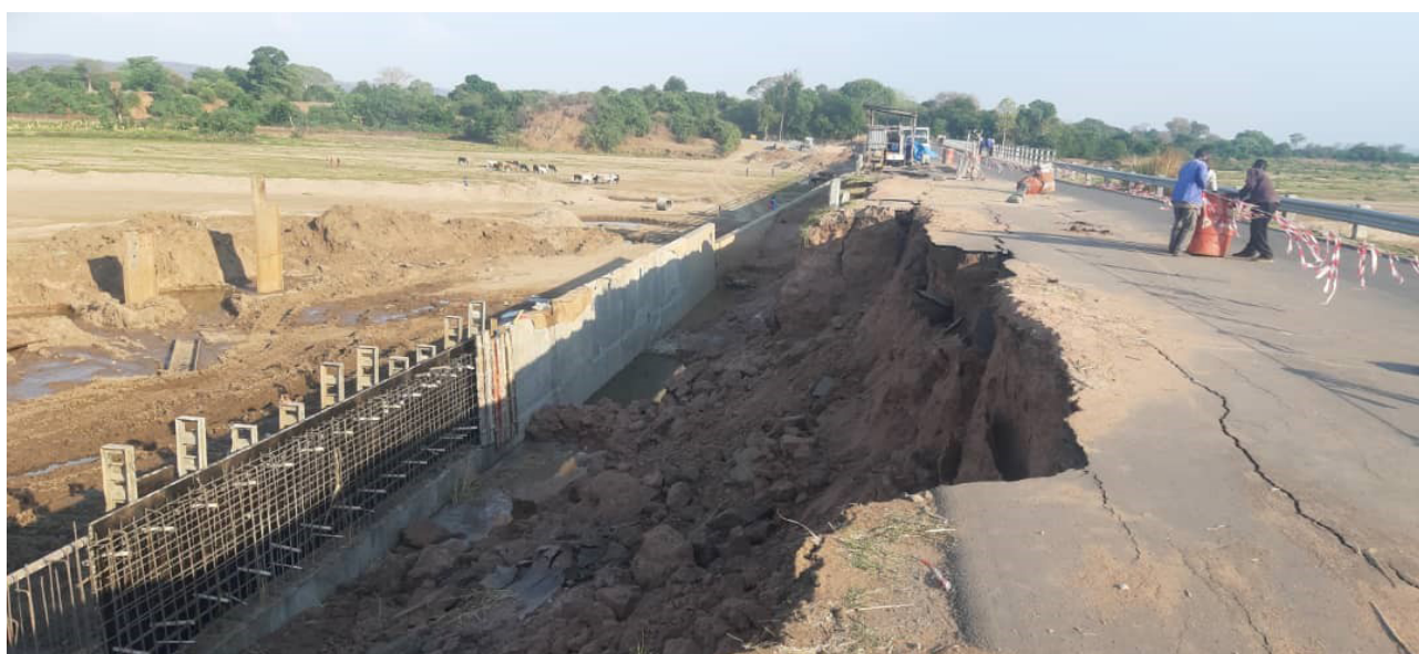
Photo 2 - Protection Works for Western Bridge Approach under Construction
