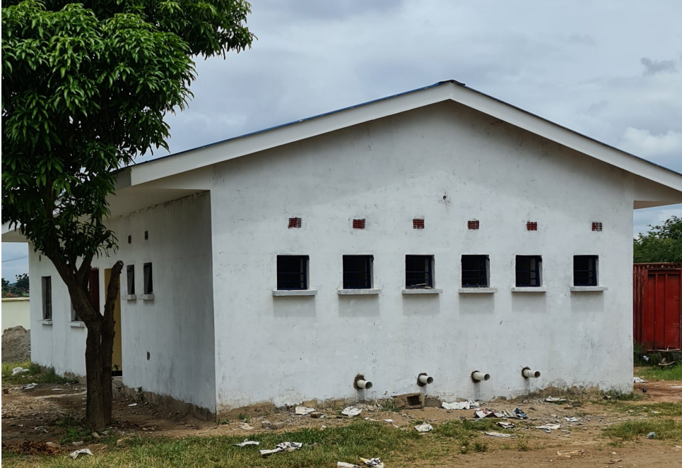
Photo 11 - Operators' Building Under Construction at Kauma WWTP
