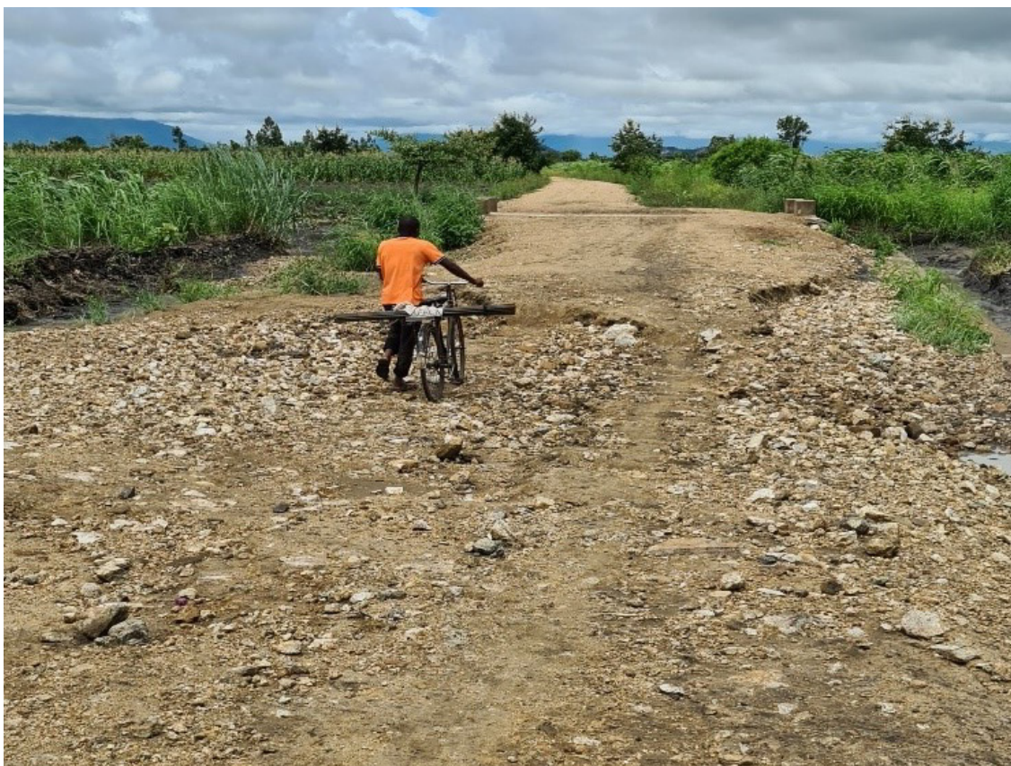
Photo 15 - Chinama Road Showing a washed Away Section.
