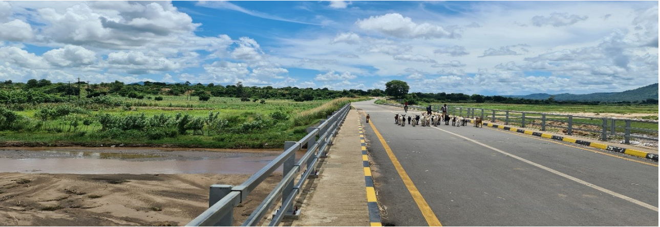
Photo 7 - Bridge under use by Community Members
