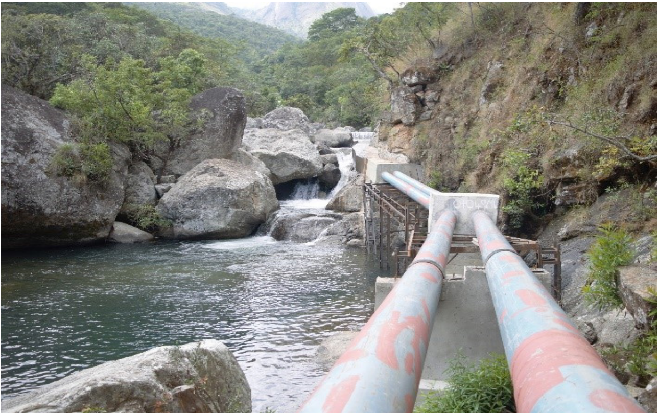
Figure 4 - Twin Gravity 350mm Diameter Pipes from Intake to Lower slopes of Mulanje Mountain
