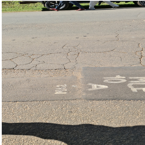
Photo 9 - Pothole Repairs under limited budget
