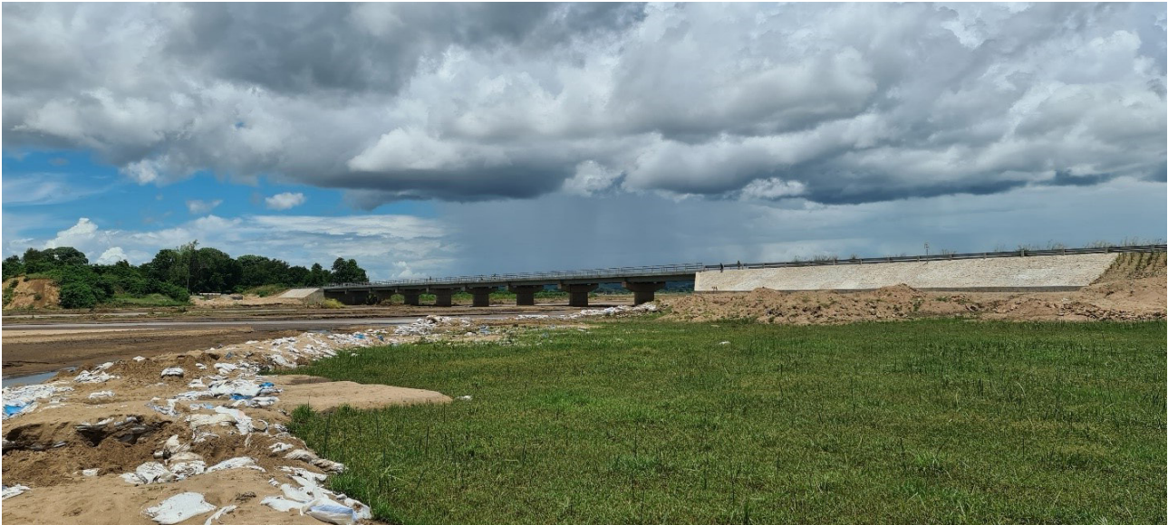
Photo 3 - Chapananga Bridge Approach Repairs Complete
