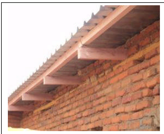
Photo MHC No. 4 – Roof timbers
