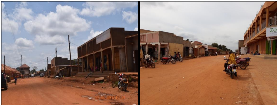
Figure 22: Road width (15m) achieved
