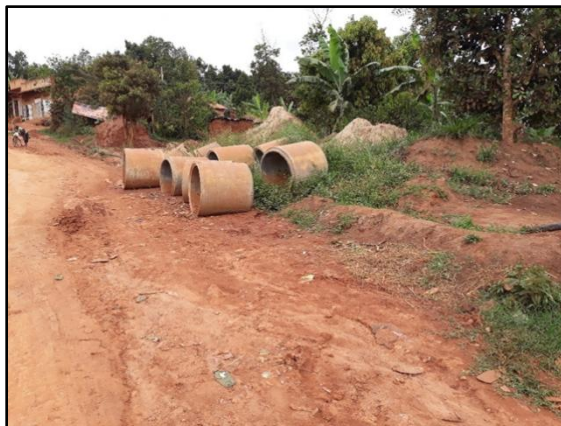
Figure 17: Poorly stored culverts on Nansanaroad
