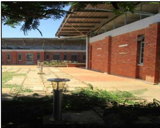
Figure 12: Solar lamp shaded by a tree at NTC Kaliro
