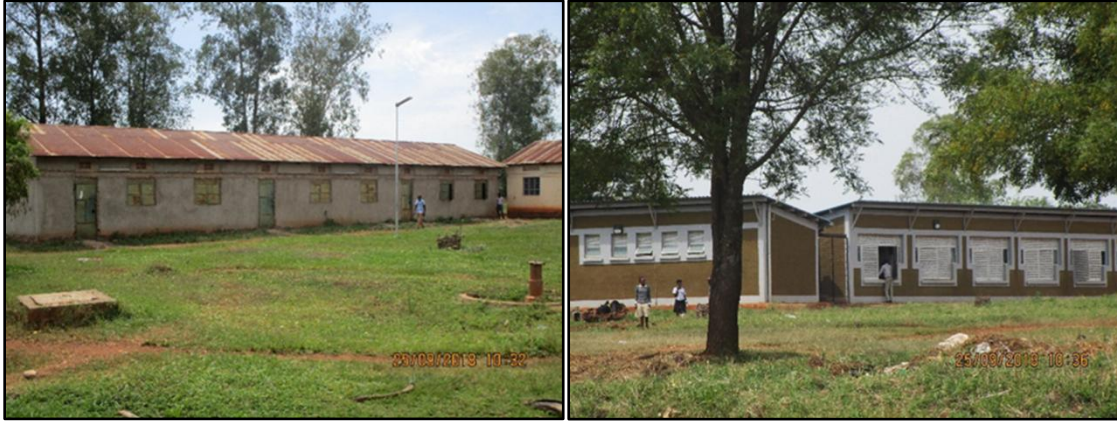
Figure 21: Improved infrastructure Old building (left) and new building (right)
