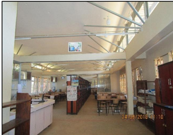
Figure 25: Effective use of natural lighting
