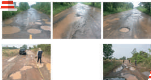
Picture illustrating damage of rural highway route no.Kor Sor Tor1-0059 Baan Moo Mon – Baan Au
