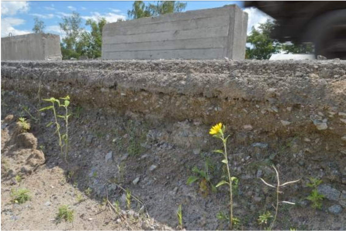
Figure 5 – Road pavement structure in Podil village, km 288+794
