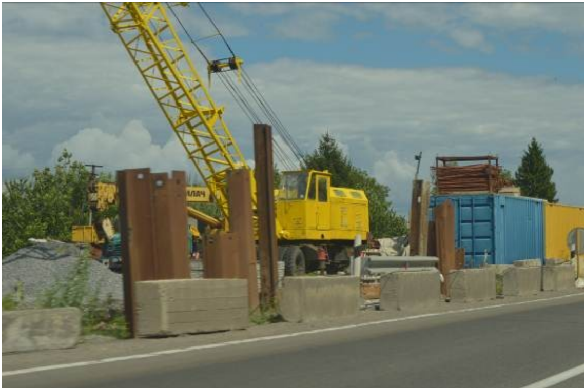
Figure 8 – Construction equipment on construction site
