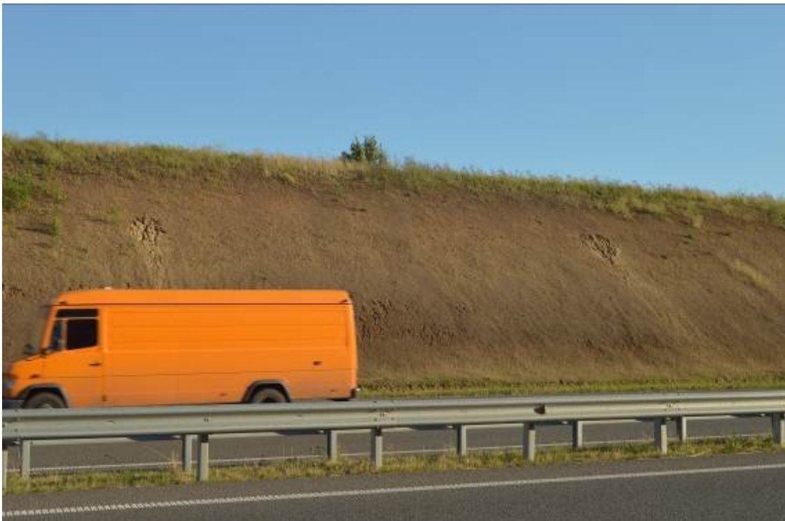
Figure 4 – Erosions, km 311
