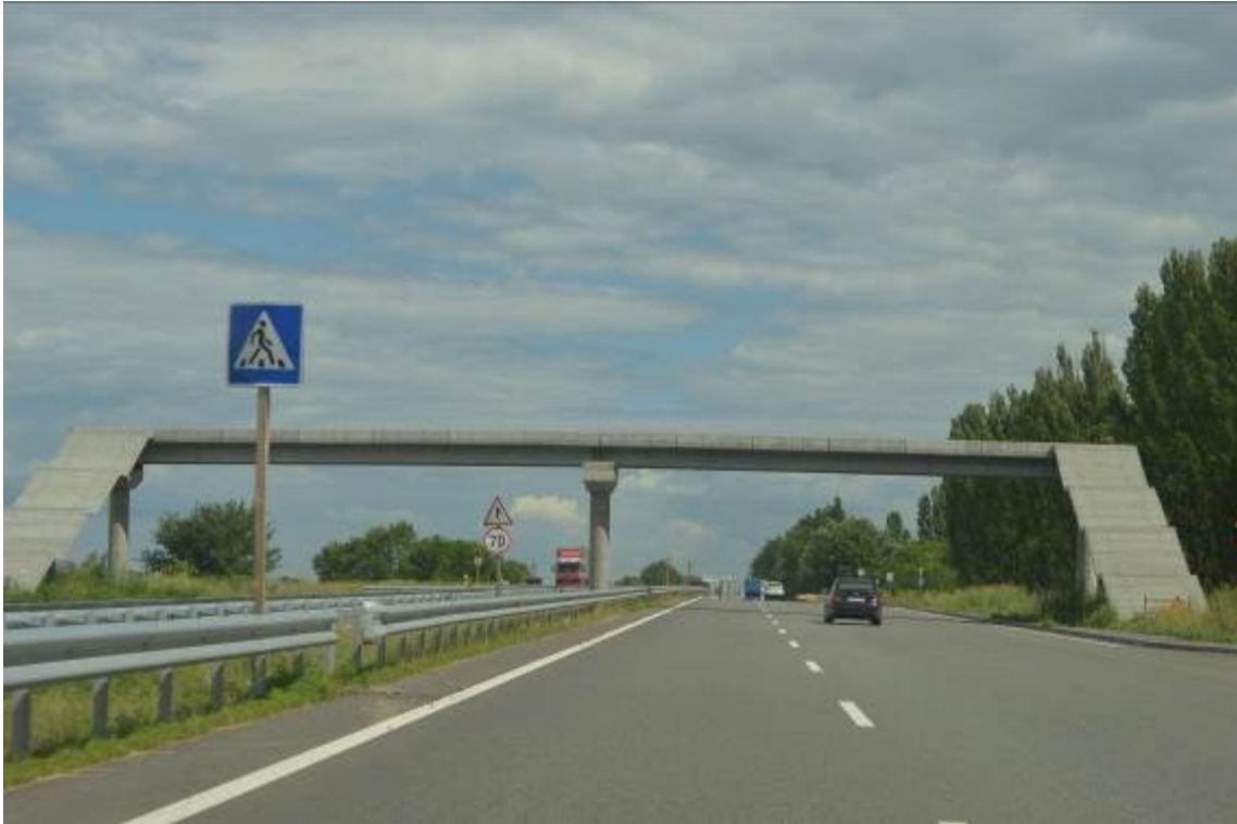
Figure 7 – Carry-over construction of overground pedestrian crossing at km 329+887 (progress \approx 60%, works are suspended)
