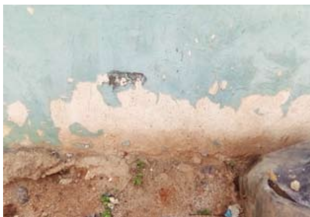
Rising damp on walls due to rising underground water by capillary action. Evidence of not considering the recommendations from the feasibility study at the design and construction stages of the project.
