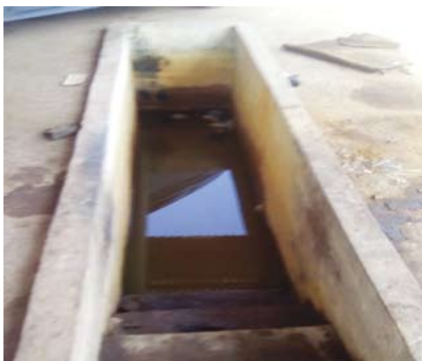
Beneficiaries of the garages are not able to use their service pits because it is always full of underground water.
