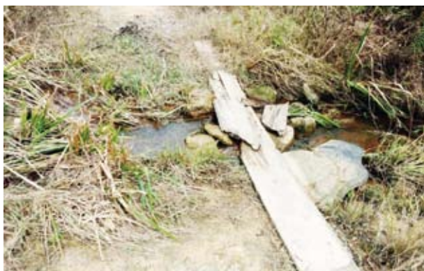
Access to the school needs improvement.
