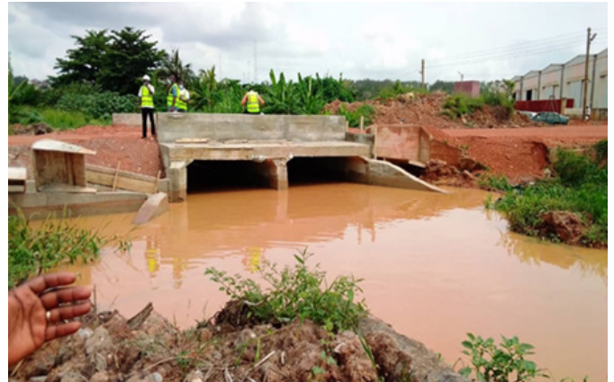
New box culvert to reduce flood risk
