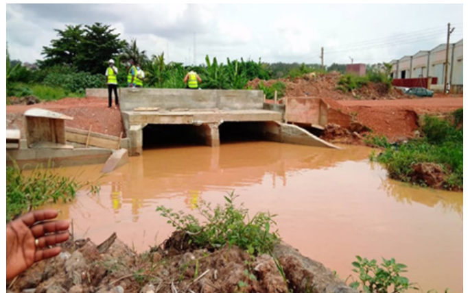
New box culvert to reduce flood risk
