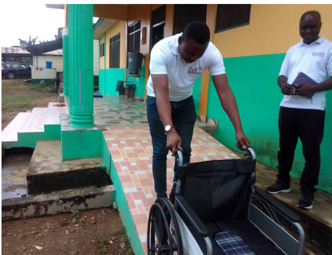
New disability ramp at the Atobiase Health Centre
