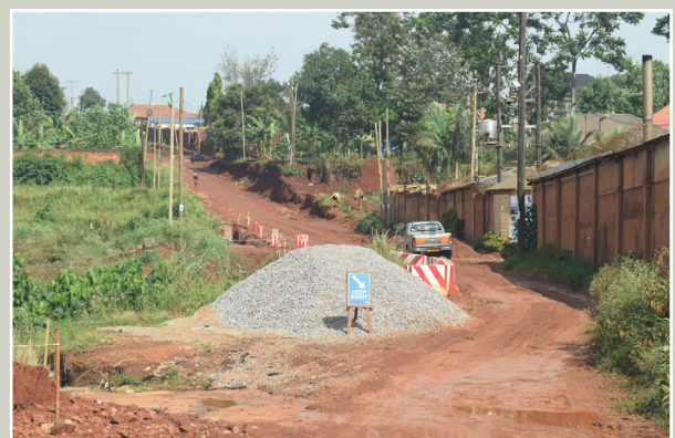
Photo taken during the construction of Katalamwa road
