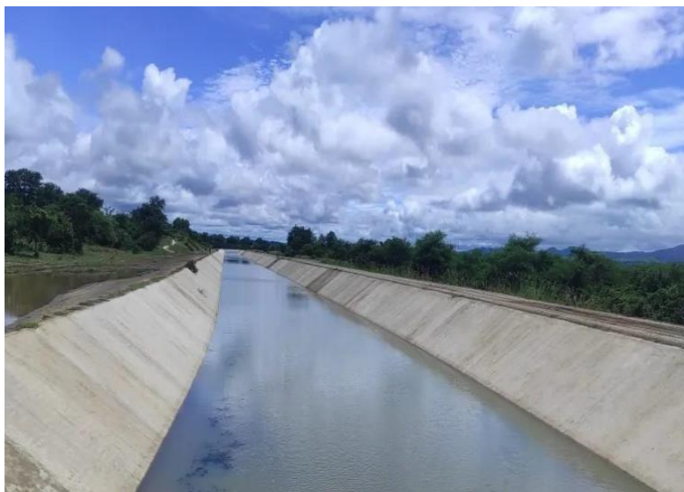
Figure 7: Shire Valley Transformation Project, Completed Section of Canal
