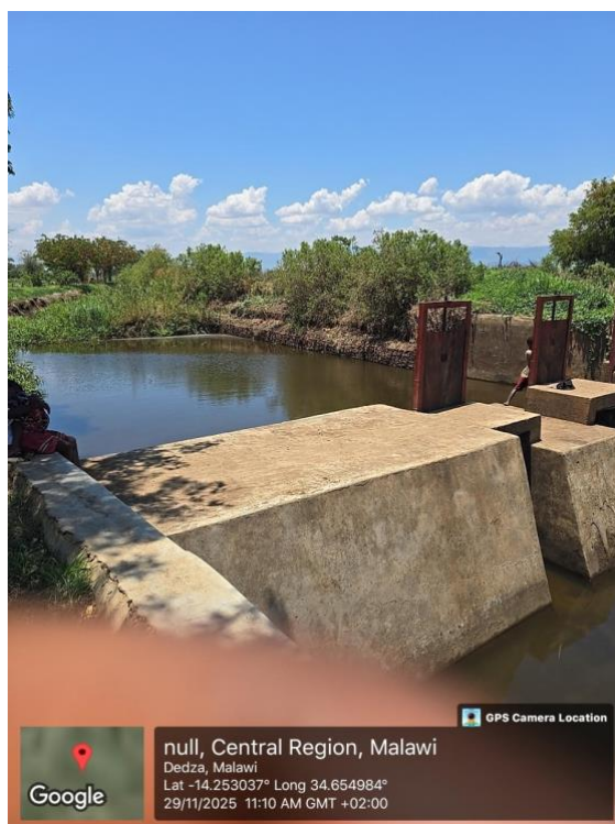
Figure 6: Intake Works at Nambuma Irrigation Scheme, Dedza District
